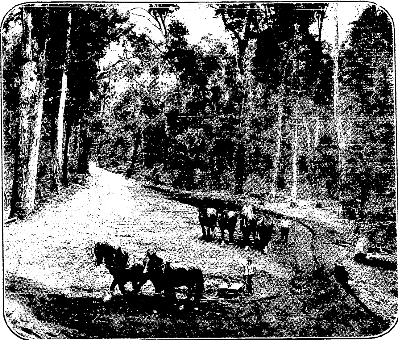
ROADMAKING IN VICTORIA.—Teams grading a road in the Dandenong Ranges, under contract with the Country Roads Board
