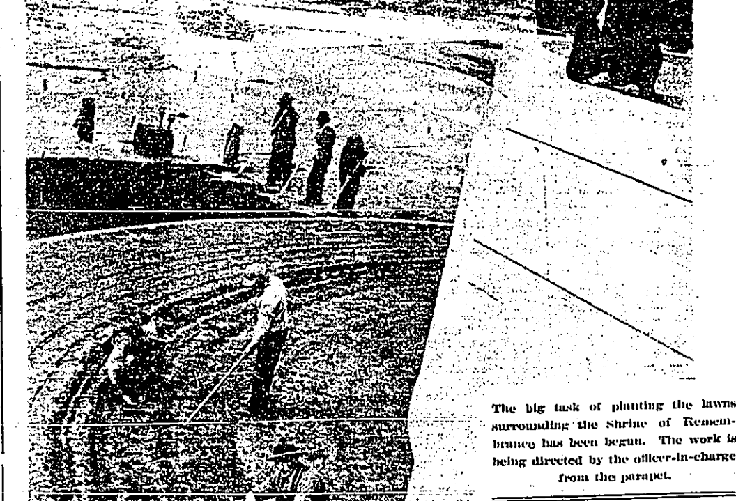
The big task of planting the lawns surrounding the Shrine of Remembrance has been begun. The work is being directed by the officer-in-charge from the parapet.
