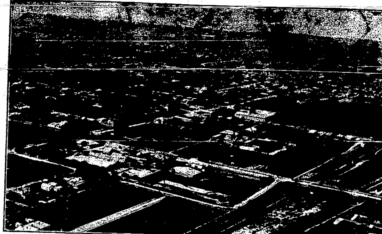
This picture, taken from an aeroplane in 1918, will give some indication of the vast strides made since those days. Many of the empty blocks shown here are now occupied by buildings. The railway is in the foreground, and on the right hand side is the Cramer Street Park. Traversing the centre on an angle (from left to right) is High Street, and alongside the Town Hall buildings is the bowling green (since transferred to a new site in Murray road.
