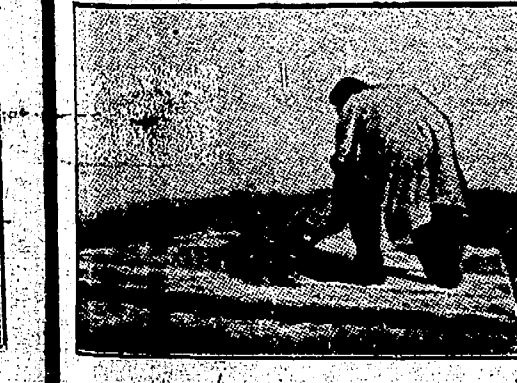
Water is then added to a depression formed in the centre of the mix. Do not use too much water.
