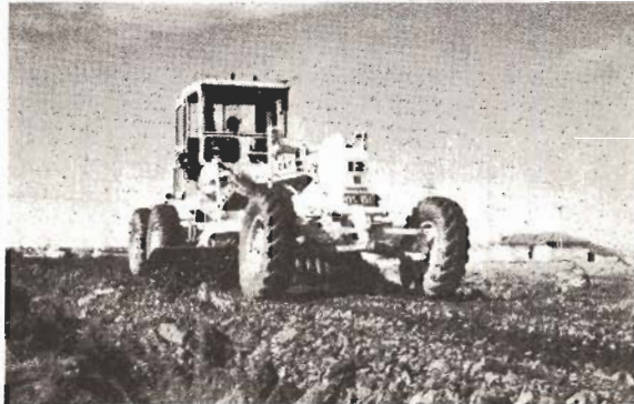
Caterpillar 12E Power Grader metalling on unmaded road.
