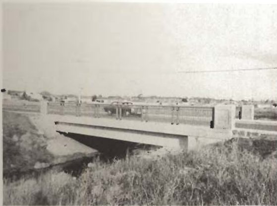
Broadhurst Ave. Bridge over Edgars Crk. Reservoir.
