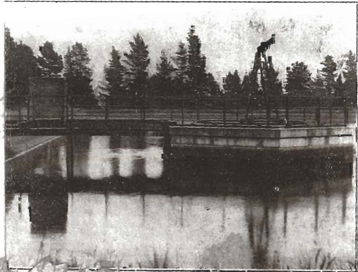
Storage, at High St., Reservoir.
